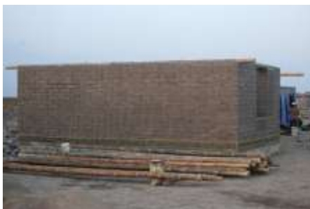
Reinforced Adobe Construction
