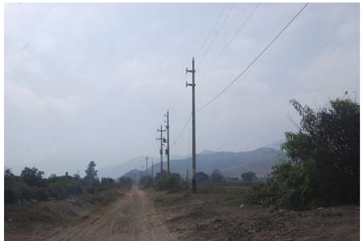
Main Roadway through Community with power lines
